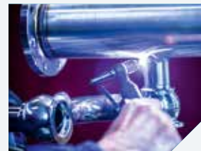
TIG welding on pigging system
