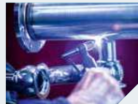
Orbital welding of a pigging station
